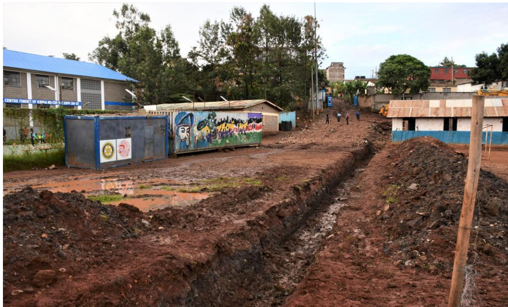
植樹地造成中の RAILA EDUCATION CENTER
